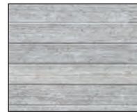
Board Formed Concrete
